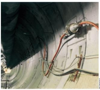
Electrical connector with a flexible 50mm<sup>2</sup>, 10kV, power feeding a full facer drilling machine from NFM Framatone in Copenhagen, Denmark
