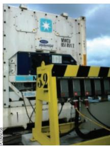
Port of Dunkerque uses Cavotec Connectors reefer point outlets for their new extension.
